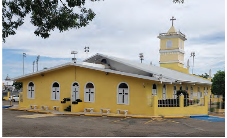
Exterior of the Sagrada Familia Parish church in Bayamón in the Archdiocese of San Juan.
